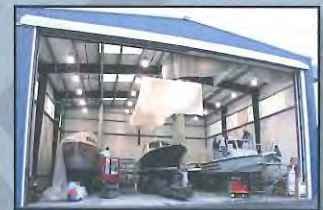
Seaview West Work Bays
